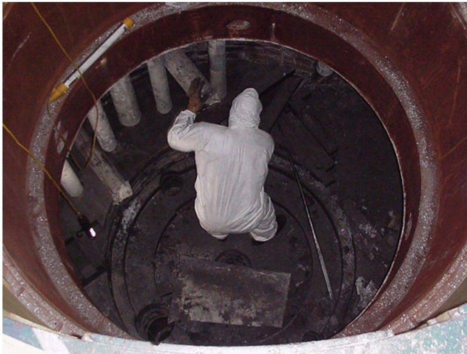
Figure 1. Graphite stringers were found to contain activated Europium because the graphite was not purified to remove the rare earth elements prior to installation.
