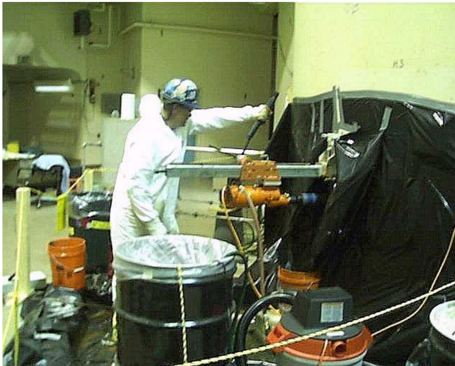
Figure 2. Intrusive sampling is best for providing meaningful characterization data about activation products in the bioshield. Modeling tools and operational data can also provide valuable information in characterizing the DD&D project.
