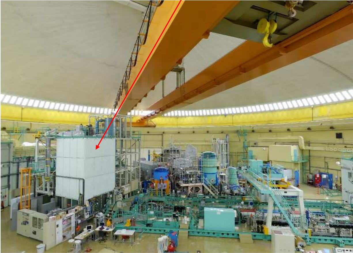
The masonry buildings inside the reactor building are in the process of being dismantled. Since these buildings house the general reactor building ventilation system, a new general ventilation system will have to be installed. (This point is the subject of another article.)
