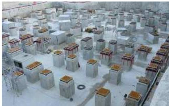
Columns bear and aseismic pads
