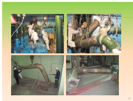
Fig 8. The part of the primary cooling system pipeline replacement
