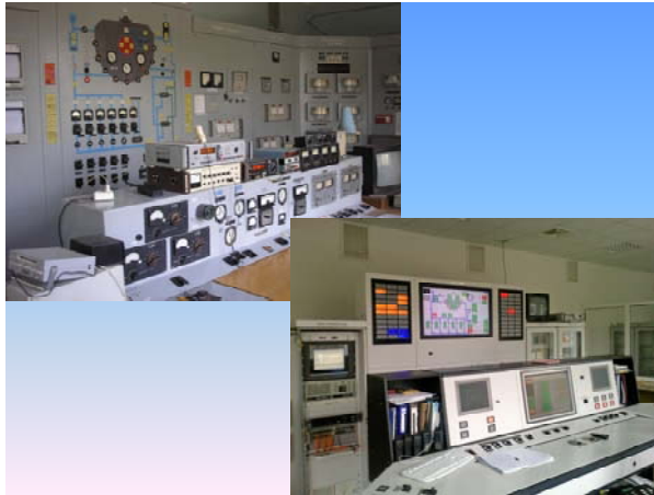
Fig 1. Reactor control room before and after refurbishment
