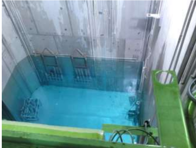
FIG. 2. Steel lining of TRR
