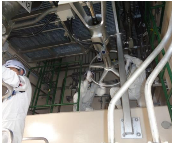
Training in manual operation of valves
