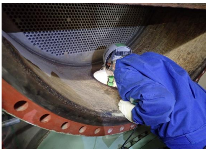
Open inspection of the heat exchanger
