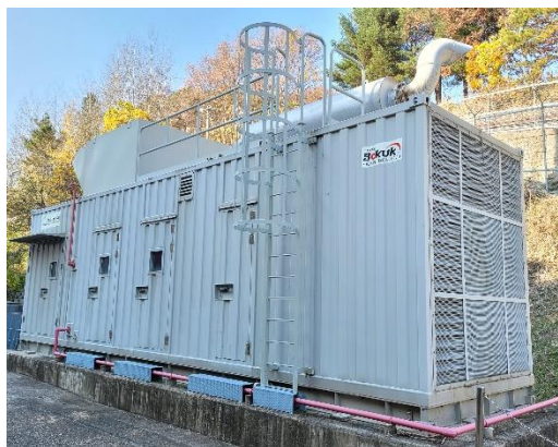
Additional emergency diesel generator
