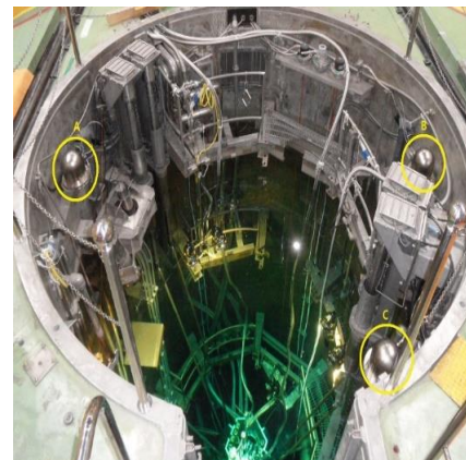
Pool Radiation Monitoring System
