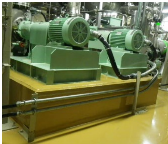
Primary coolant auxiliary pump (I secure the height of the foundation)
