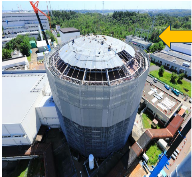
Reinforcement work on the roof of the reactor building
