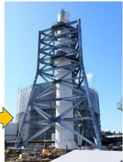
Reinforcement work of exhaust stack
