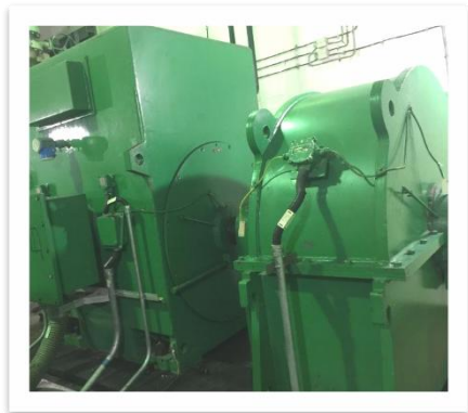
Main pump with flywheel
