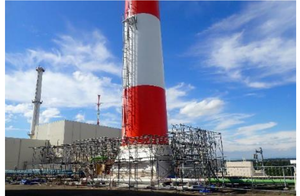
Anti-seismic Reinforcement on the Main Stack
