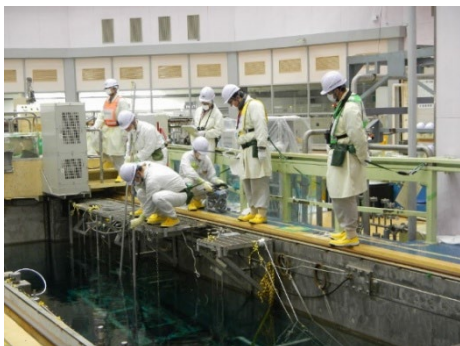
Storage work after removal of control rods
