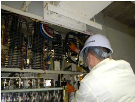
Disconnecting power cable
