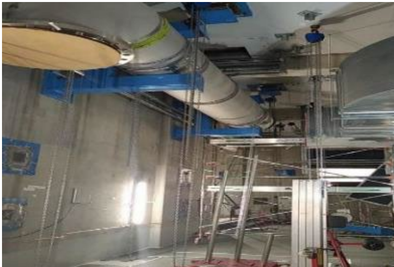
Installation of supports and pipes in the cooling circuit building
