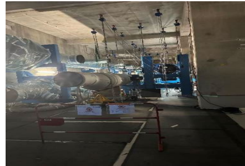
Installation of supports and pipes in the cooling circuit building
