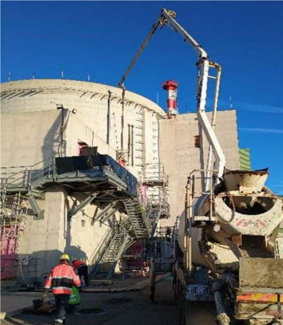
Concrete pouring in Safeguards building
