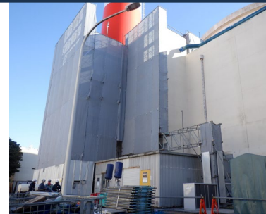
Seismic reinforcement on the exhaust stacks
